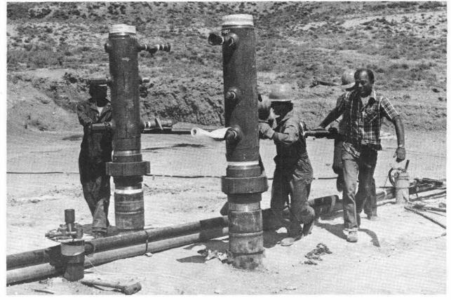
JOHN TALBOT (1132), right, helps a drilling crew install explosive well head loaders at the site of an oil shale rubblizing experiment. Both hydrofracture techniques and explosive slurry were used to rubblize an underground oil shale formation.
